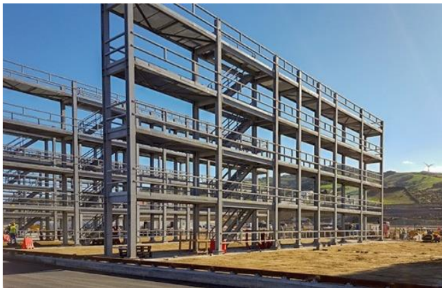
Figure 3-1: A permanent scaffolding that attaches to the exterior of a high bay system with built in stairs that acts as a cheap way a human can access a container on a higher level.
