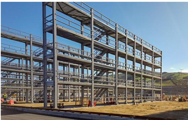
A permanent scaffolding that attaches to the exterior of a high bay system with built in stairs that act as a joint accessway.
